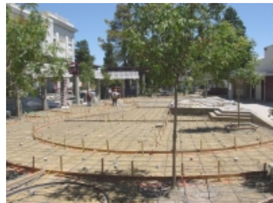
Quad under construction
