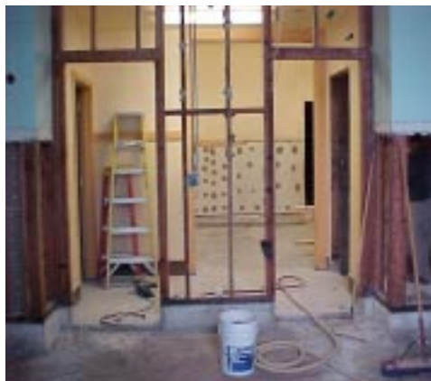
Remodeling of toilet rooms
