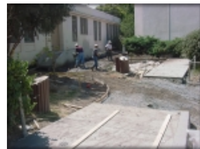
New sidewalks being installed
