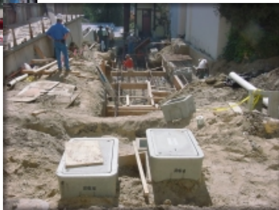
Excavation for ramp between math building and science building
