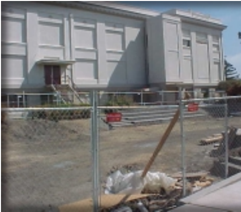
Quad area renovation
