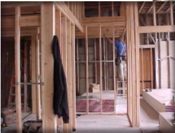
Framing for new student counseling offices
