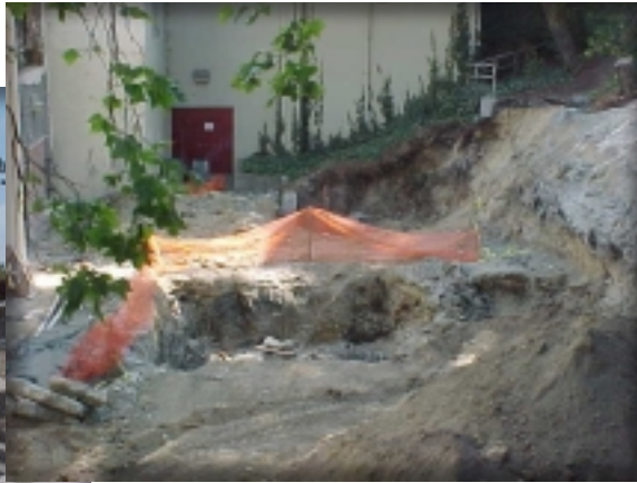
Excavation for elevator to gym
