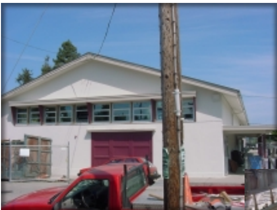
New windows for shop building
