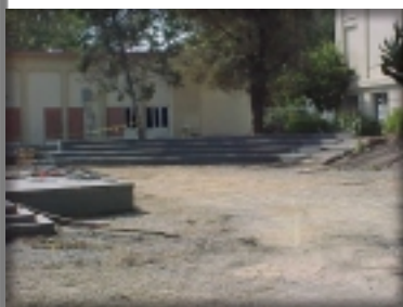
Old concrete is removed to make way for new quad area
