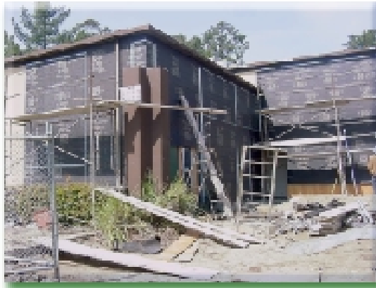
Exterior finishes to Humanities Building
