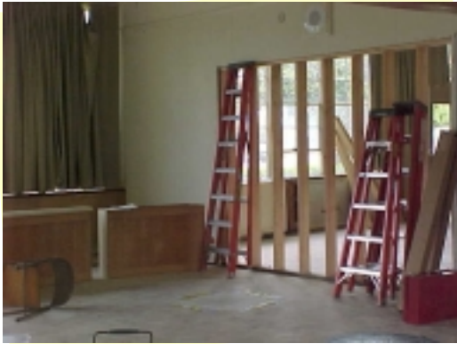
Classroom under construction
