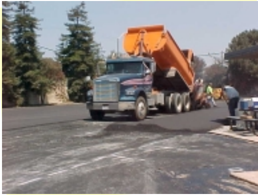
New pavement for parking lot
