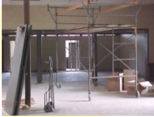
Library under construction
