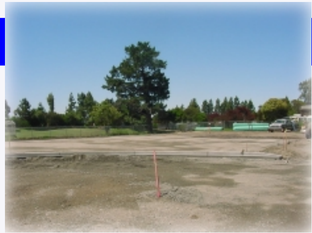
Preparing the site
