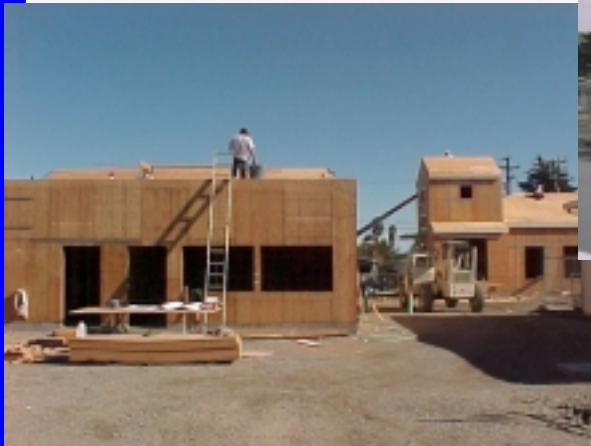
Above and left: Wood sheathing applied to framing of independent studies building
