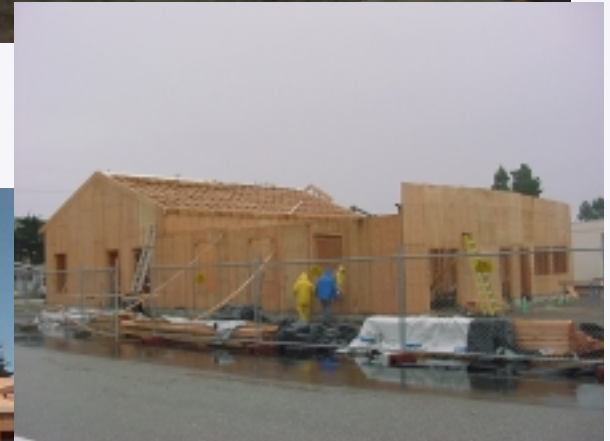
Above and left: Wood sheathing applied to framing of independent studies building
